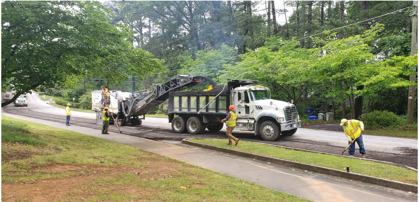
Resurfacing picture: The City of Tucker's 2020 paving contract which SEI's Senior Inspector Mike Lehner oversaw.
